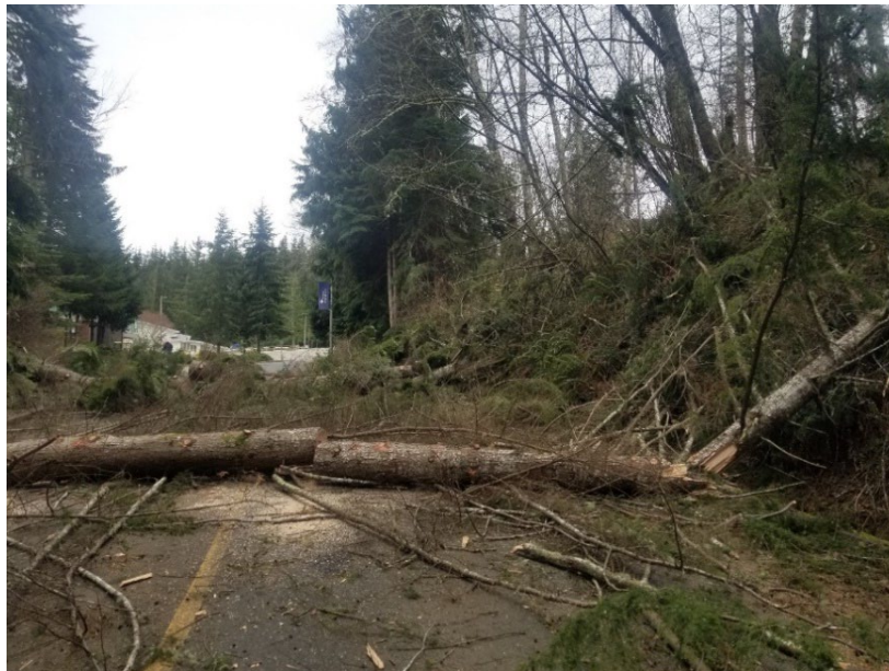
Figure 4 Grays Harbor College Road blocked by trees and woody debris.
